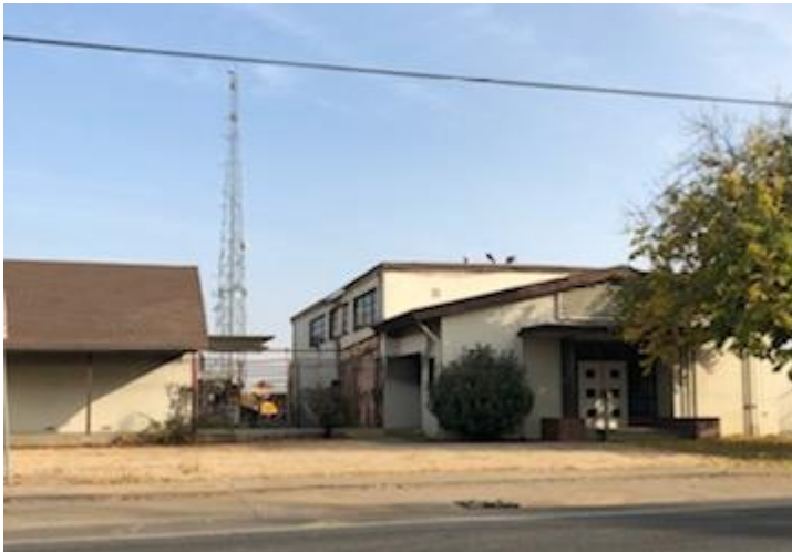
FIGURE 9: Transportation Office Building 2. Building to be removed. Transportation offices to be relocated to San Joaquin Street facility.
