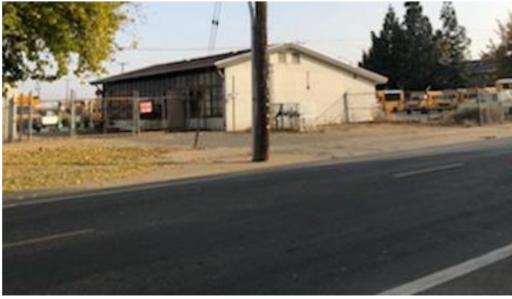
FIGURE 10: Transportation Office Building 3 (bus maintenance facility). Building to be removed. Transportation offices to be relocated to San Joaquin Street facility.
