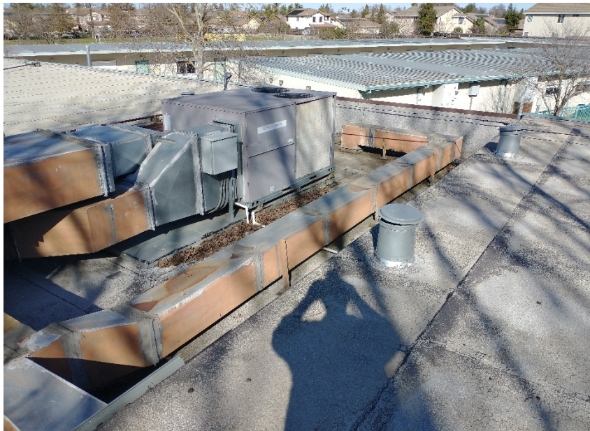
Administration Building Roof & HVAC
