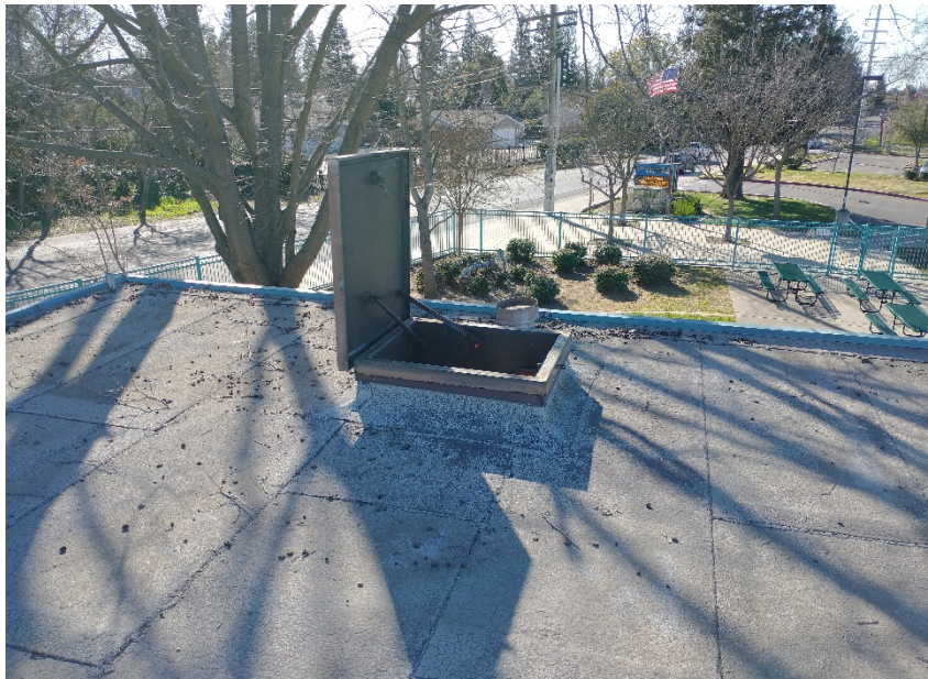
Administration Building Roof
