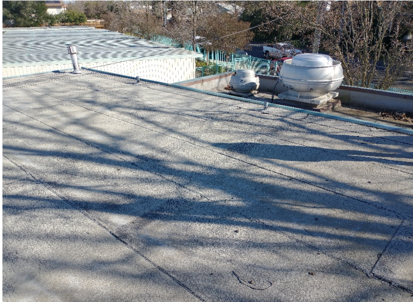
Administration Building Roof
