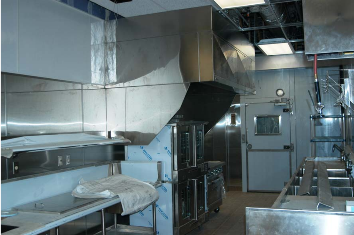
Kitchen in Multipurpose Building
