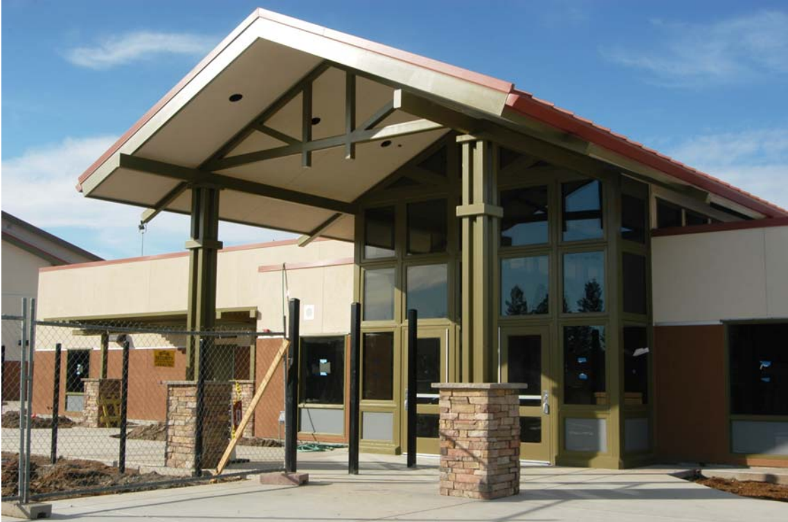
Building A - Administration
