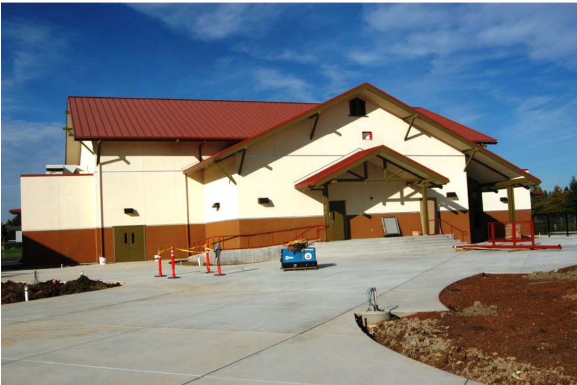
Bldg E - Multipurpose
