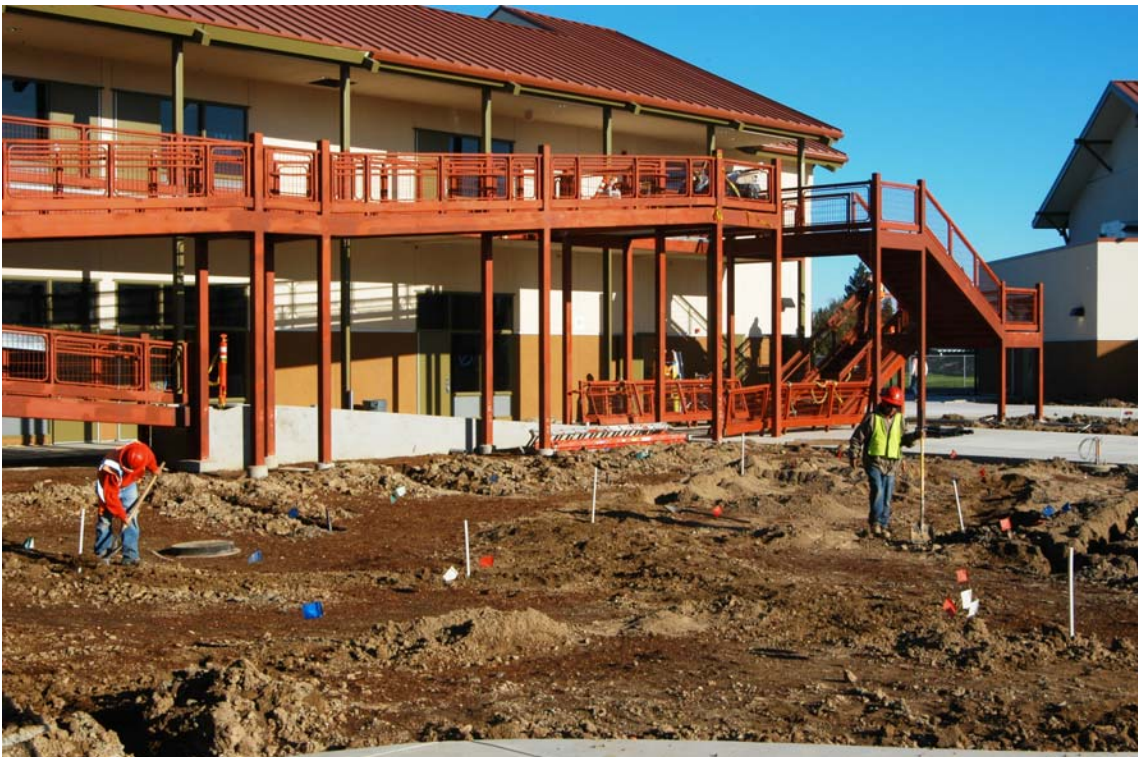
Installing Landscaping in Courtyard
