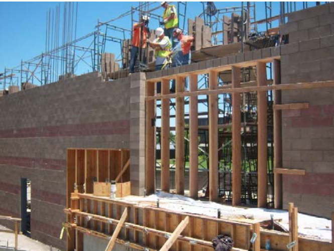
Installing Masonry Reinforcing
