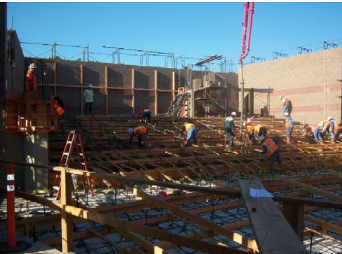
Placing Concrete Steps at Assembly
