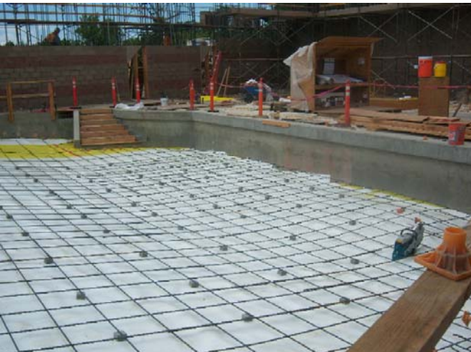
Waterproofing at Lower Assembly
