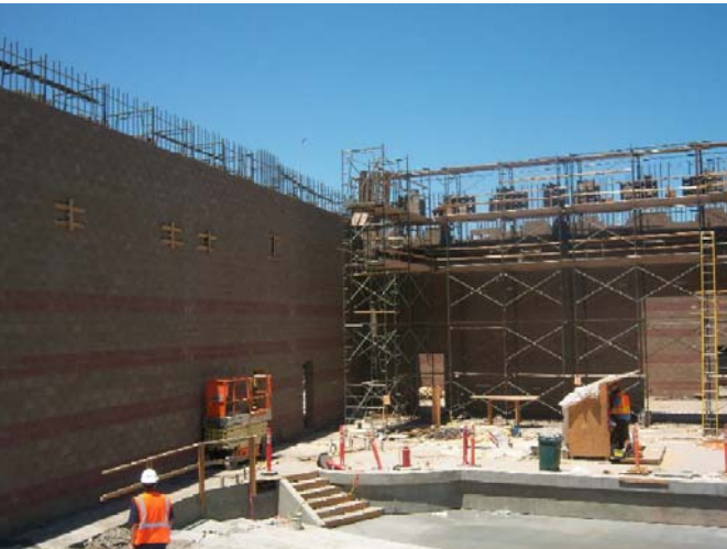
Masonry Block Installation Ongoing
