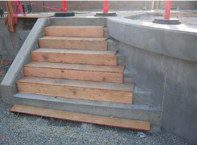
Stairs at Stage
