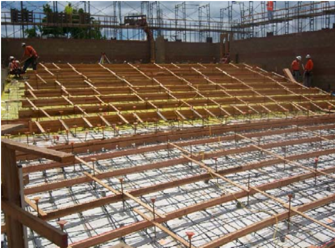
Formwork at Assembly
