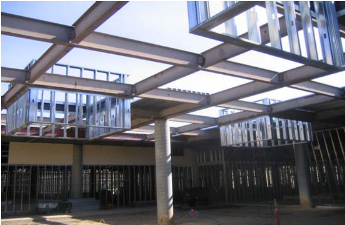
Skylight Framing in Courtyard.
