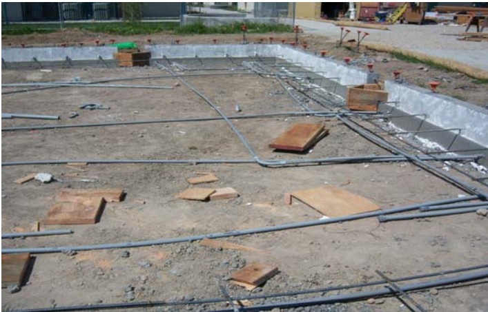
Under slab electrical in progress.
