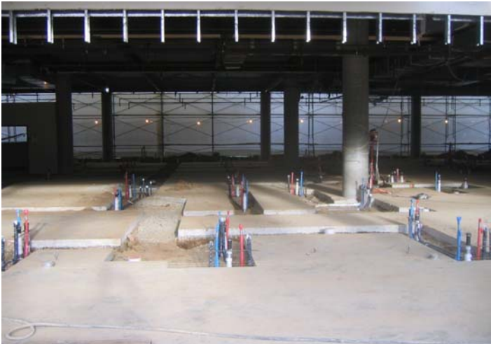
Under slab plumbing at Science classrooms.
