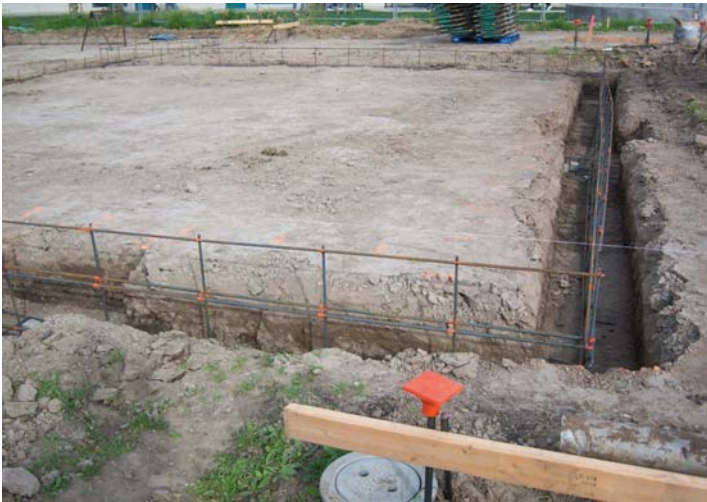
Rebar placement for building foundation.
