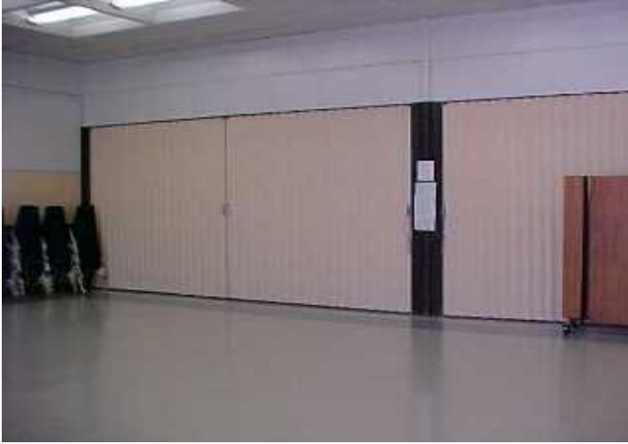
New accordion doors between Cafeteria and Kitchen.
