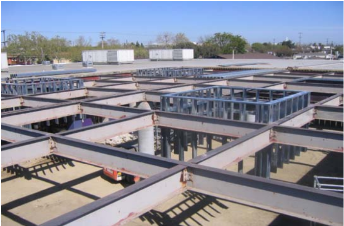
Courtyard From Above.
