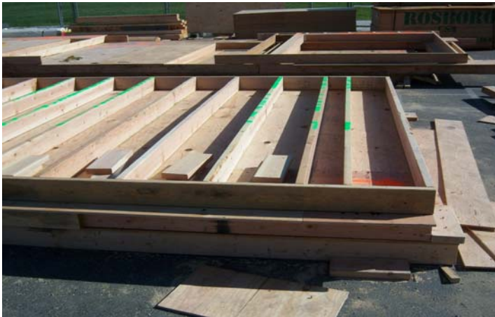
Preparation for wall framing.
