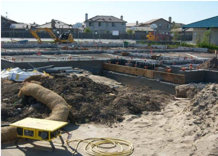
Overview of Building E foundation.
