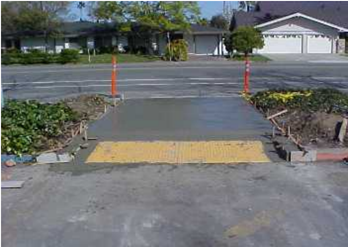
New ADA ramp with truncated domes.
