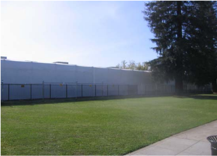
Shrink wrap on the exterior of the West Wing.
