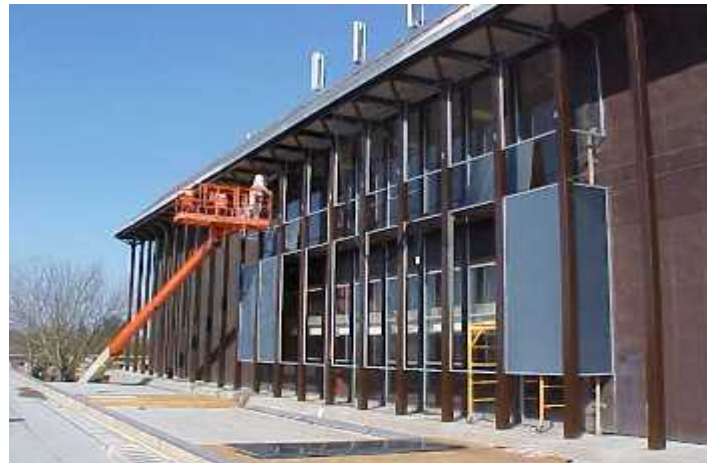
Removal of old plexiglass sunshades.
