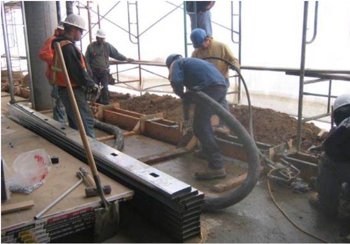
Perimeter Footings Poured on East Side.
