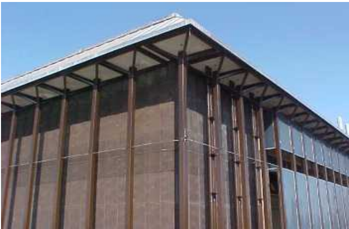
Installation of new bird deterrent netting.
