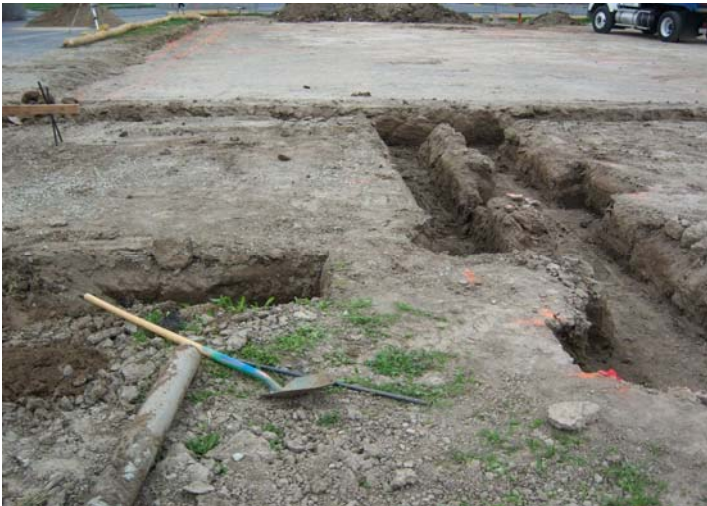
Trenching for building foundation.
