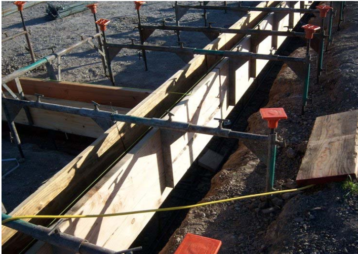
Formwork in place for foundation.
