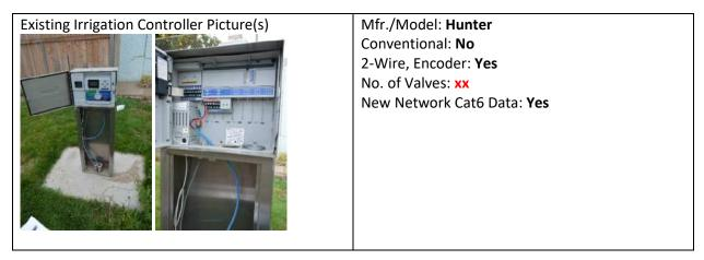
Description: Existing Hunter conventional controller to be replaced. Reuse existing underground cabling. Clip and re-terminate all lead ends to new controller and existing valves. Install new Cat6 network cable to controller from existing network rack IDF - location approx. 200'.
