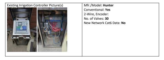
Description: Existing Hunter conventional controller to be replaced. Reuse existing underground cabling. Clip and re-terminate all lead ends to new controller and existing valves. Install new Cat6 network cable to controller from portable building, room 69 network rack IDF 1.07 - location approx. 150'.
