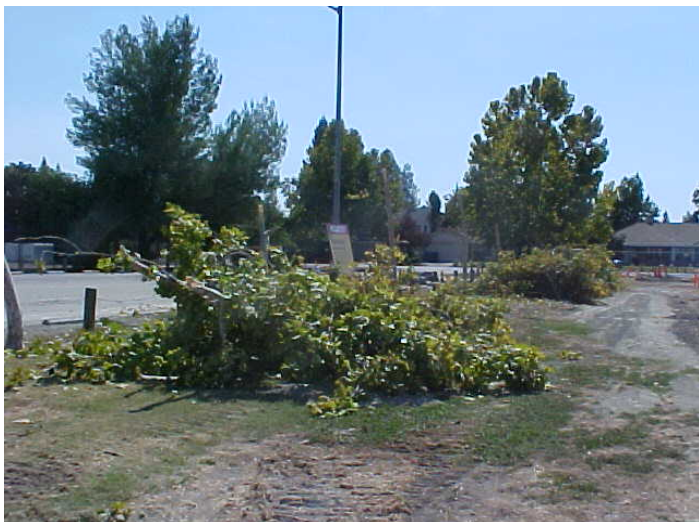
Demolition of Trees on the City Parcel
