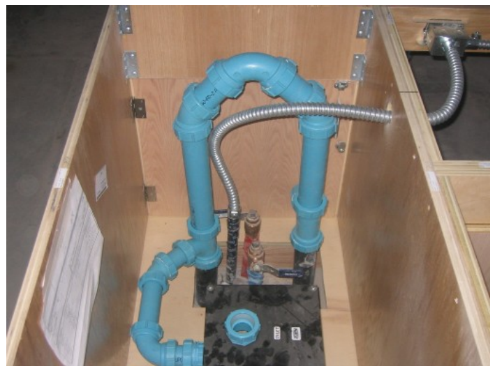
Acid Resistant Pipes and Tank in Casework
