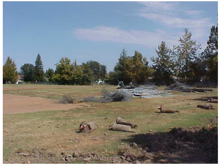
Demolition of the Baseball Backstops and Fencing
