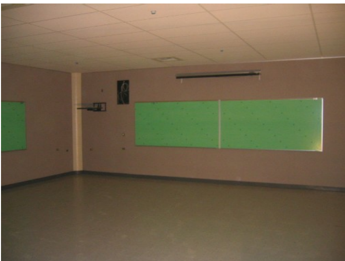
Classroom Minus Electrical and Fire Sprinkler Trims
