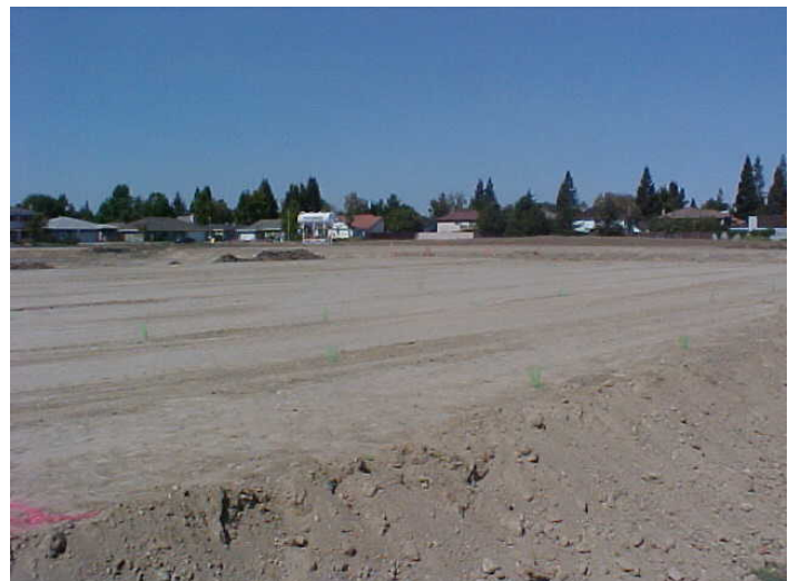
Imported Fill to Construct the Building Pads
