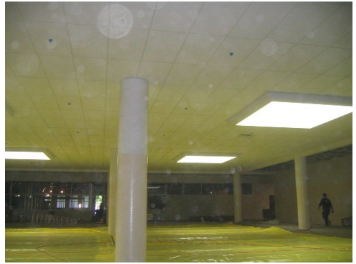
Vapor Barrier and Ceiling Tiles Installed in Courtyard
