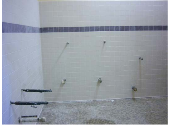
Phase 6 Restrooms – Ceramic Tile Overlay
