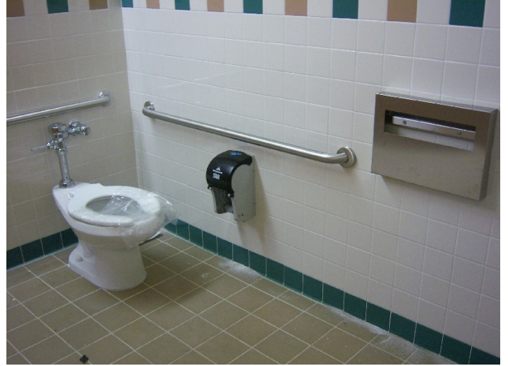
Newly Installed Restroom Fixtures and Accessories
