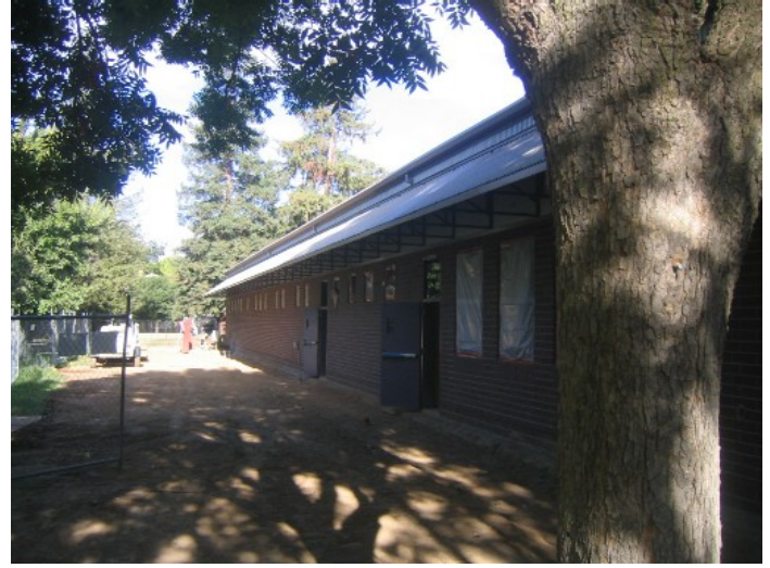
Awnings & Thin Brick Complete on South Wall
