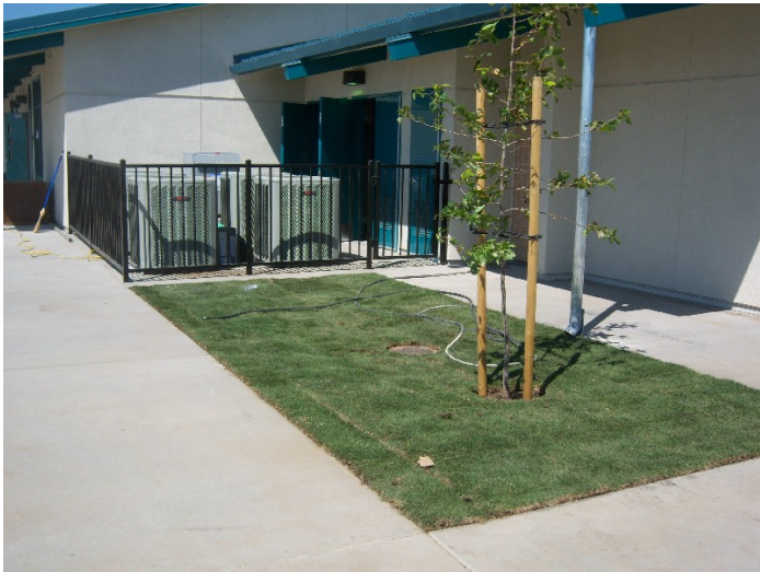
New Landscaping and Service Yard
