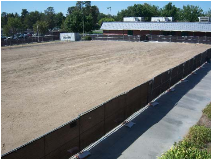
Fencing with Screen Around Theater Building Pad
