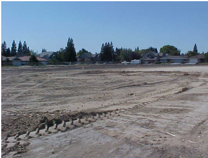
Subgrade for the South Parking Lot
