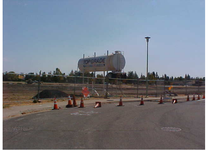
Water Tower Set Up for Grading Operation
