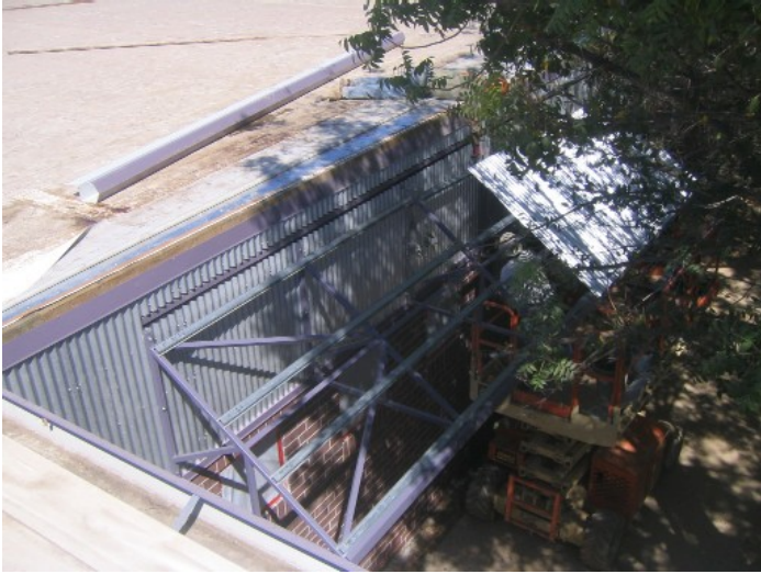
Installing Final Awning Truss
