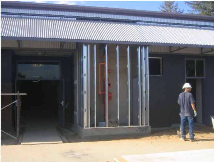
Fire and Gas Riser Room is Framed
