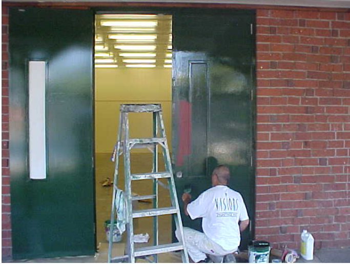
Exterior Door Painting
