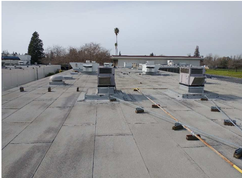
Roof of Northeast Classroom Building Showing Roof Jacks and Curbs
