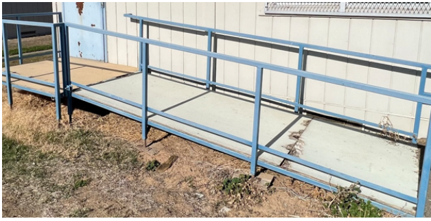
Plywood Replaced on 1 Ramp & 1 Stairs
