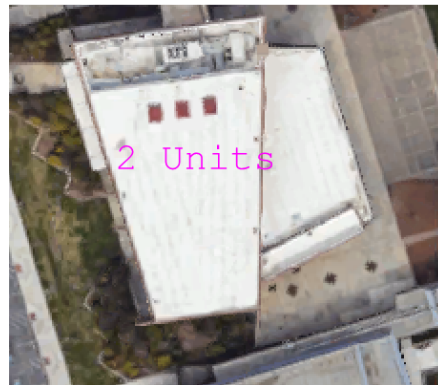
N Wing with its 2 RTU's
