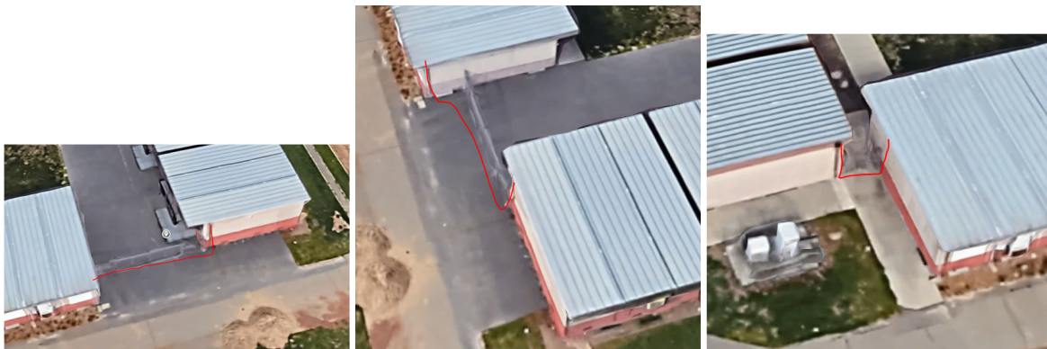
Expected pathway between T wing portable gap to get all of T wing on single loytec
