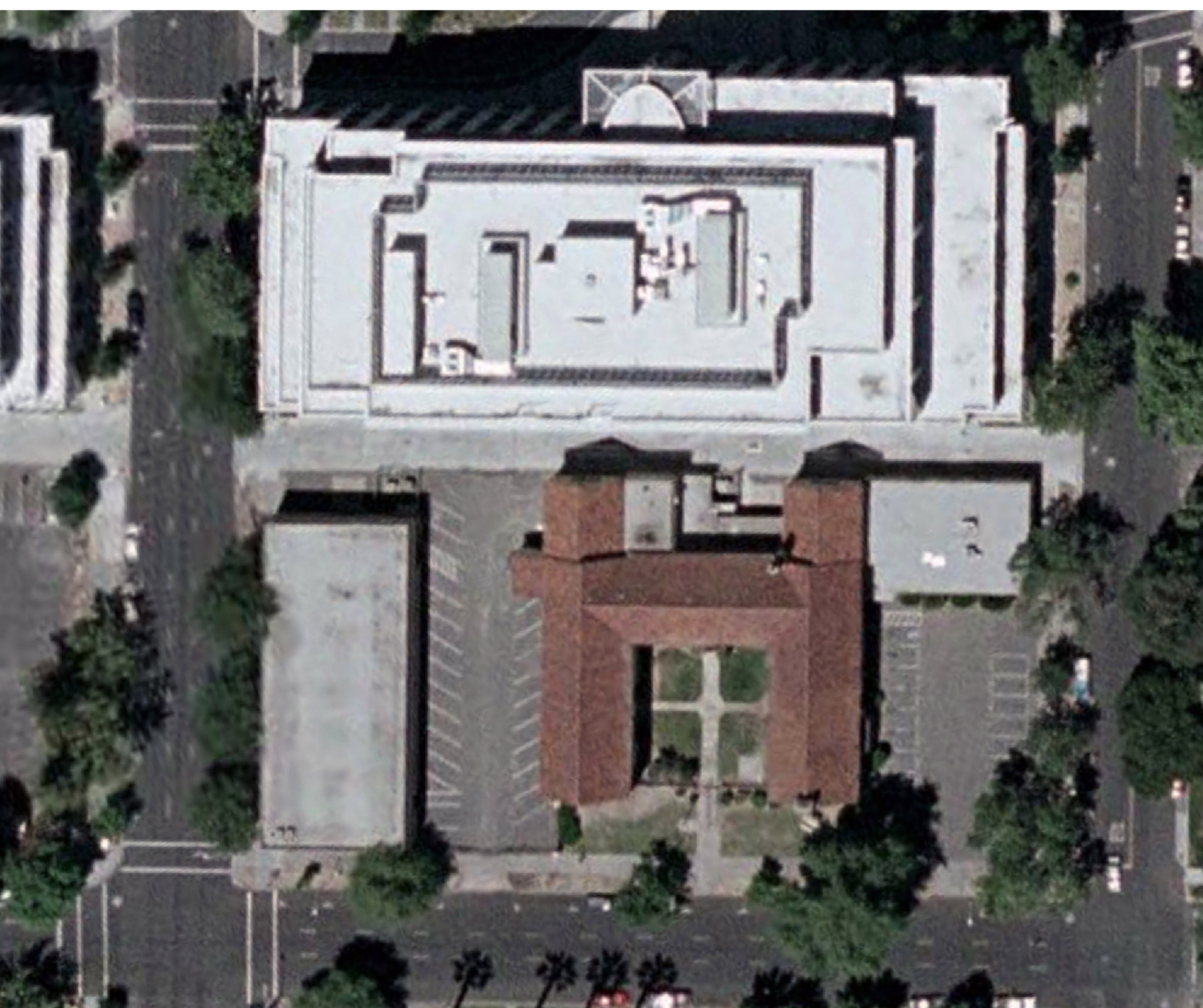
16th and N St. Admin Complex
