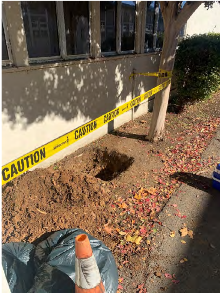
Photograph of IDW excavation to remove lead-impacted soil at location B-16
