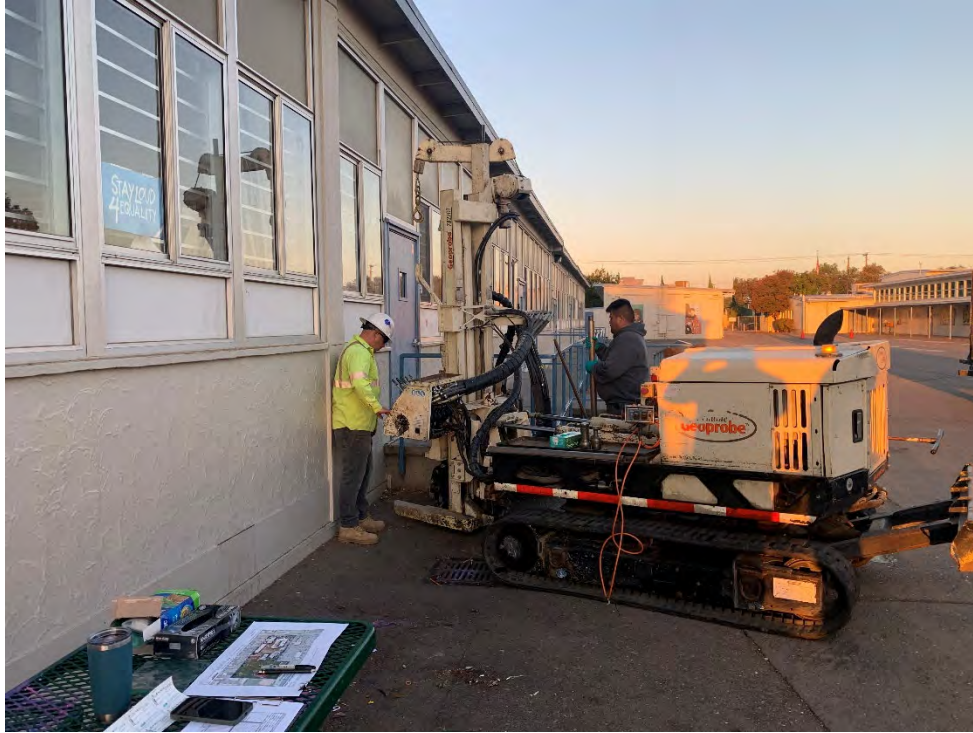
Photograph of Geoprobe drill rig obtaining soil sample next to main school building
