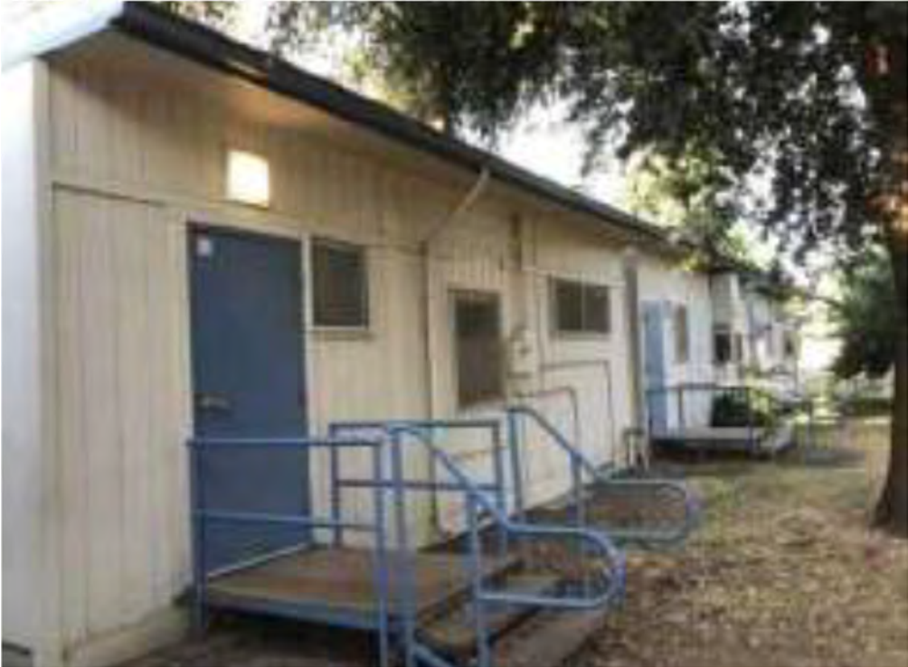
Portable classrooms east of main permanent buildings
