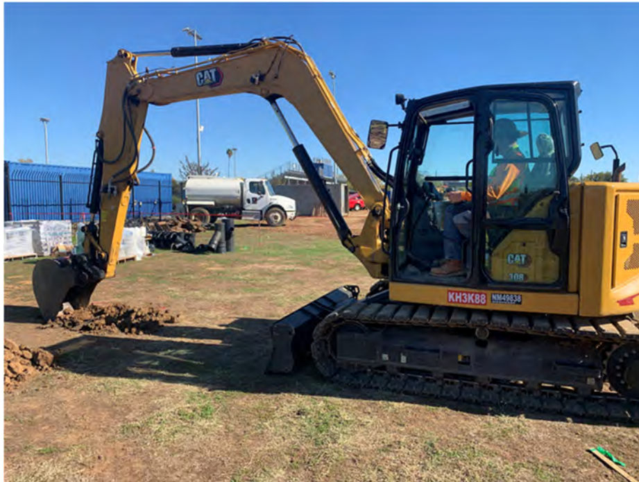
Excavation of lead-impacted soil with backhoe at location B-56
