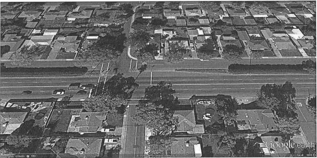
FIGURE 7: Fruitridge Road and Helen Way. Signalized Intersection with cross walks. Helen Way connects with Irvin Way and Harte Way as a route from C.P. Huntington Elementary to Hollywood Park Elementary.
