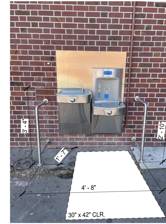
NOTE: DRINKING FOUNTAIN IMAGES ARE SHOWN FOR VISUAL REFERENCE. DIMENSIONS AND CLEARANCES HAVE BEEN CONFIRMED PER THIS DETAIL.
