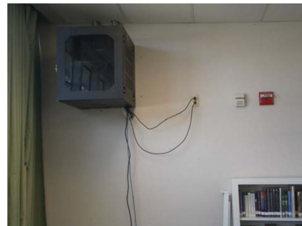
Indoor Environmental Quality IDF makes loud motor sounds that disturbs the students and staff.
