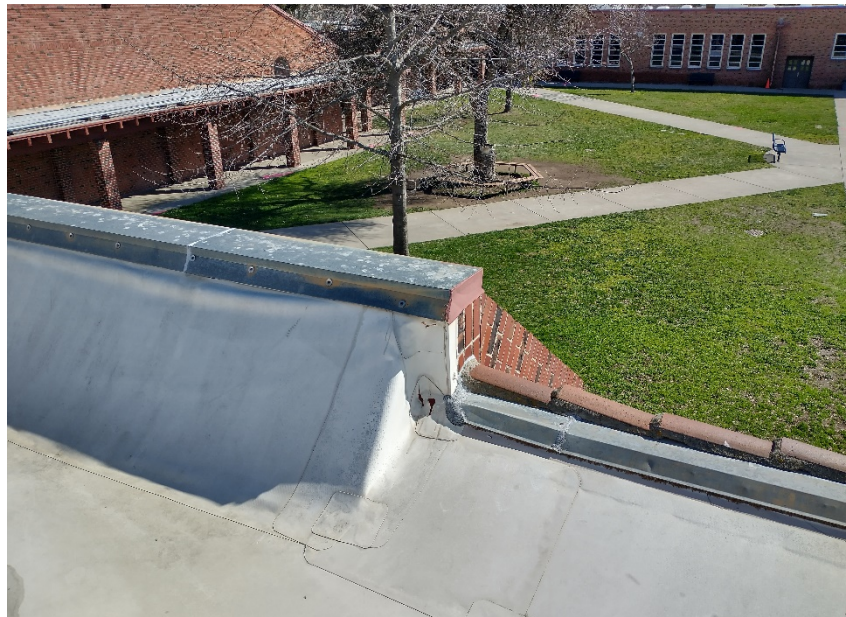
Main Building Parapet Wall with Flashing and Clay Roofing Tile Adjacent
