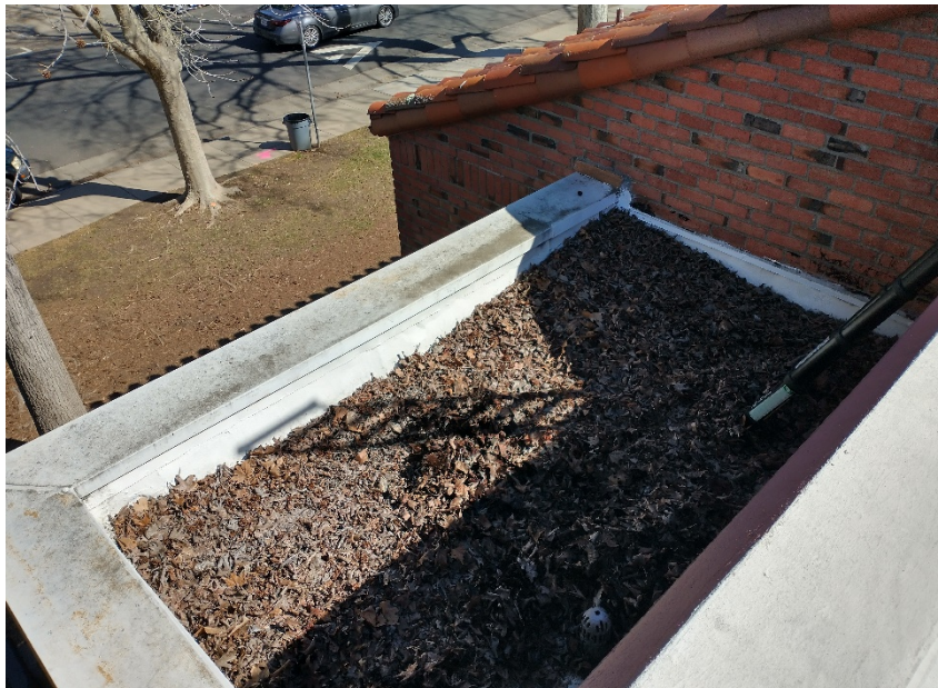
East Building North Side Lower Roof with Asphaltic Roofing
