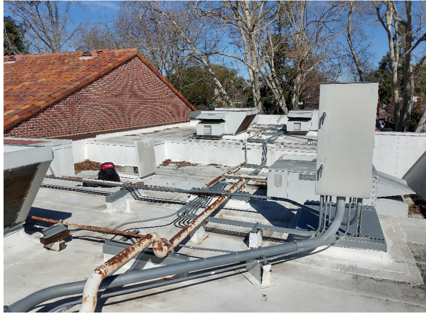
East Building with Asphaltic Roofing
