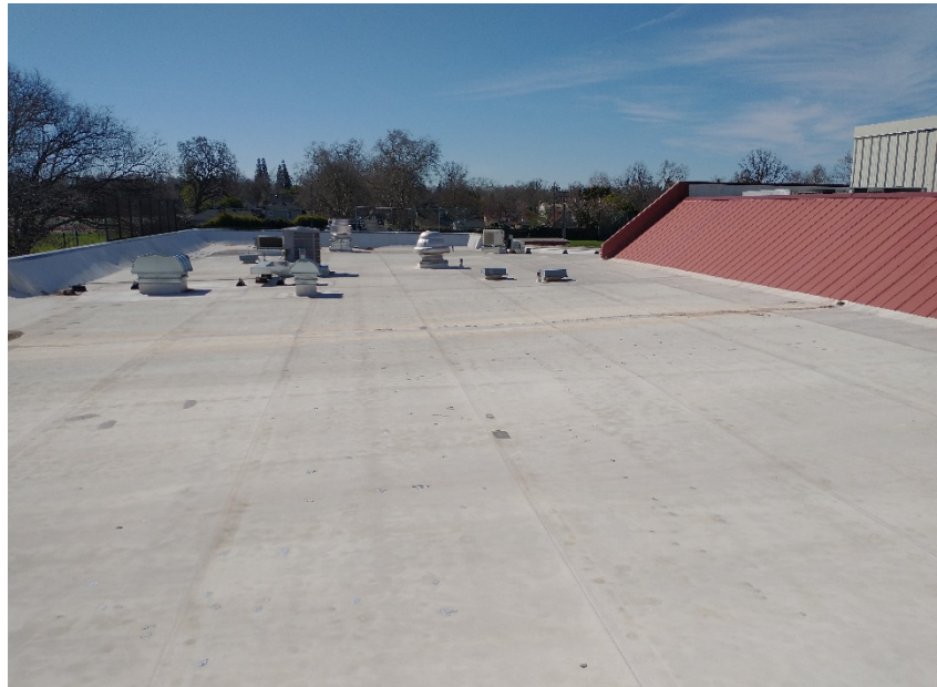
Main Building Single Ply Membrane Roofing
