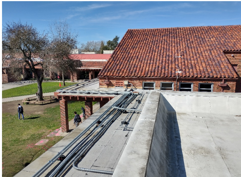
East Building Covered Walkways with Asphaltic Roofing
