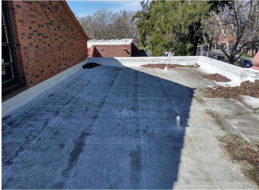
East Building North Side with Asphaltic Roofing
