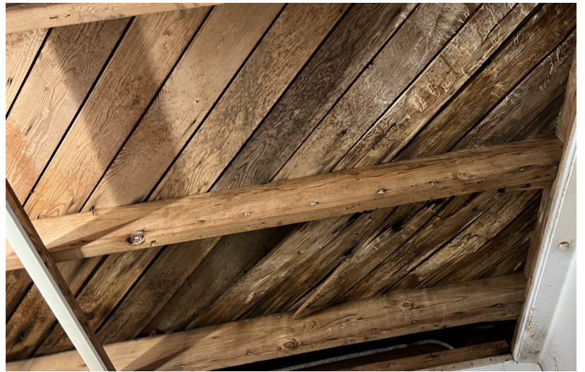
Roof Substrate Repair
