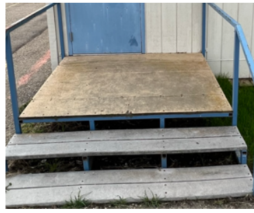
Plywood Replaced on 1 Ramp & 1 Stairs
