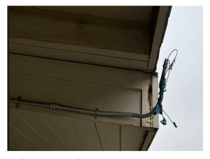
Open Electrical Conduit with Exposed Wires
